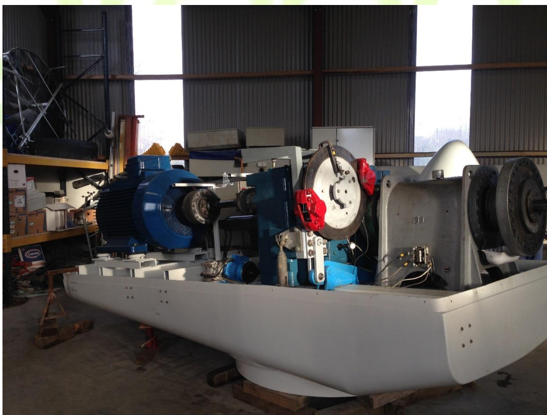
Rebuilding of V27/29
